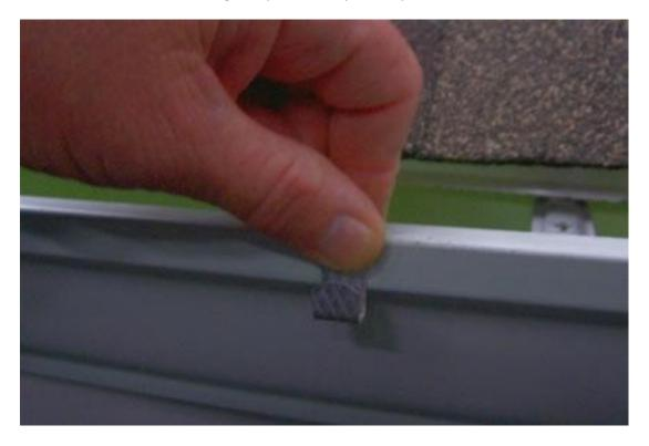
Or squeeze with pliers to permanently lock in place
